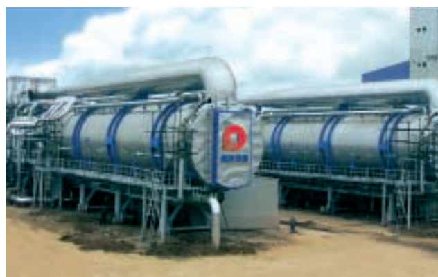
Desalting facility of Huanghua Power
