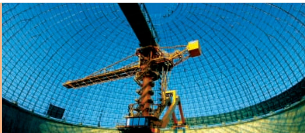
Spherical coal depot in construction
